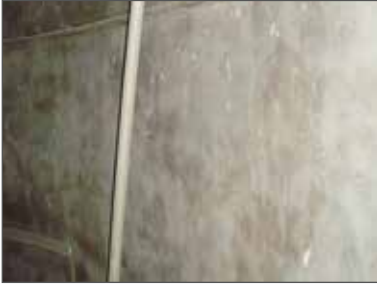
下地処理 / After Pre-Treatment
