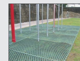
施工直後 After application
