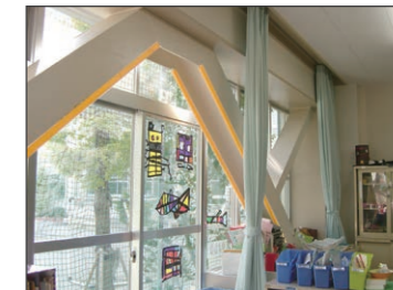
耐震補強工事のH鋼 Earthquake-resistant steel structure
