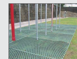
施工直後 After application
