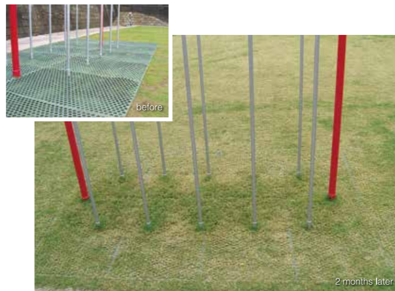
芝保護マット(校庭緑地化工事後の芝に施工) Truf-Protection Mat (for School Ground Greening)
